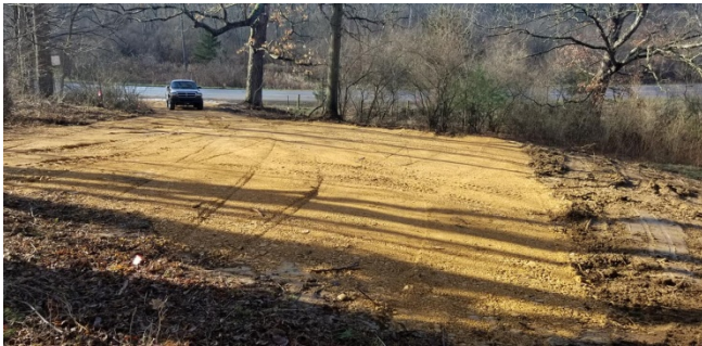
Parking area is roughed out and graded at Penn Aqua (photo by Karen Bange)
