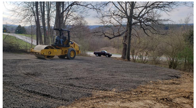
Gravel down and roller action at Penn Aqua (photo by Karen Bange)
