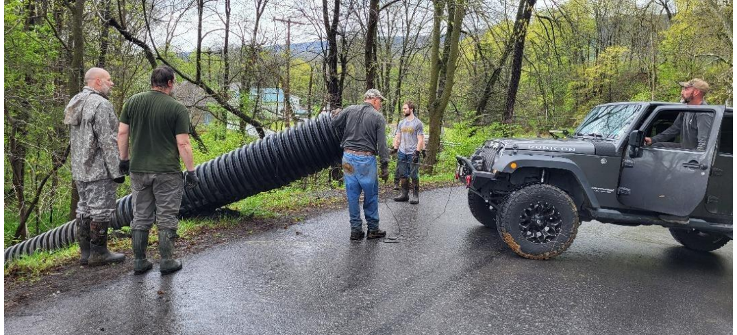
Hauling the culvert pipe up the steep slope using Jesse's winch (photo by Karen Bange)
